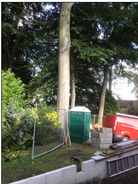
Plate 1: T1 (in foreground), T2 and T3
