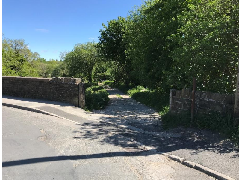
Photograph 2 – Existing Access Track
