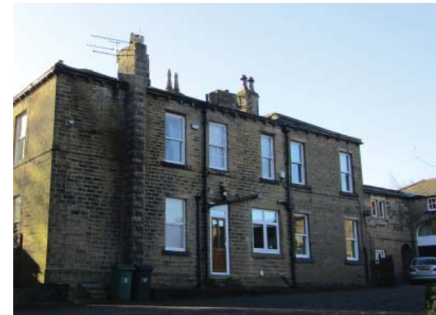
Rear Elevation with down pipes and altered projecting chimney stack.
