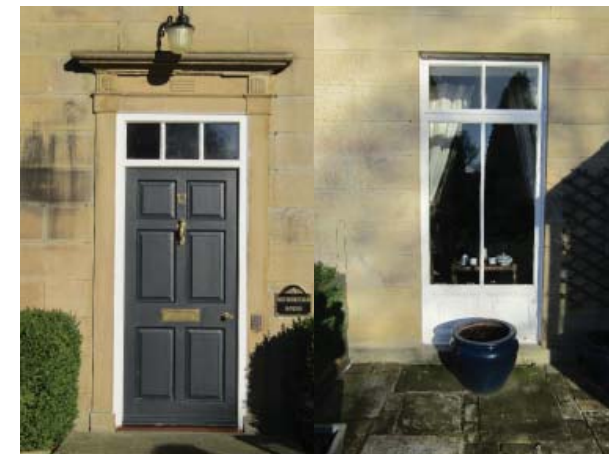
Well proportioned doors and windows. Door with modest decoration typical of the style.
