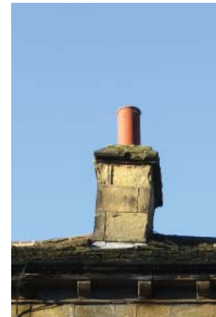
Chimney leaning with apparent damage to roof. Additional chimney Stack.
