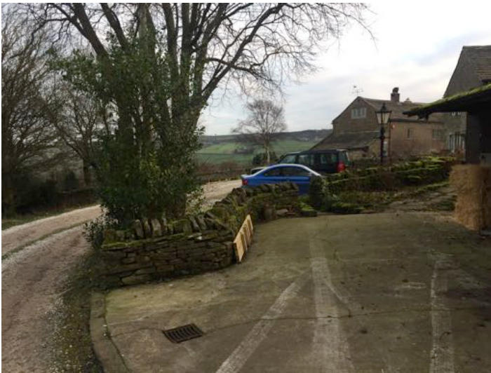
2. Front of stable block
