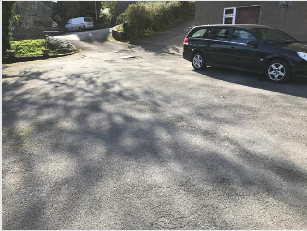
Figure 6. Concrete hardstanding within the centre of the site.
