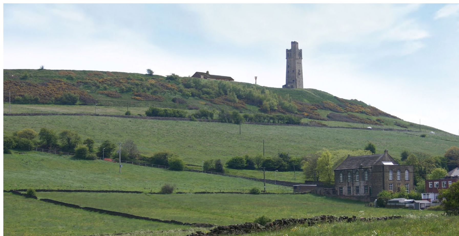
Photomontage Viewpoint Location 2 - As existing (top) with proposed image below for comparison
