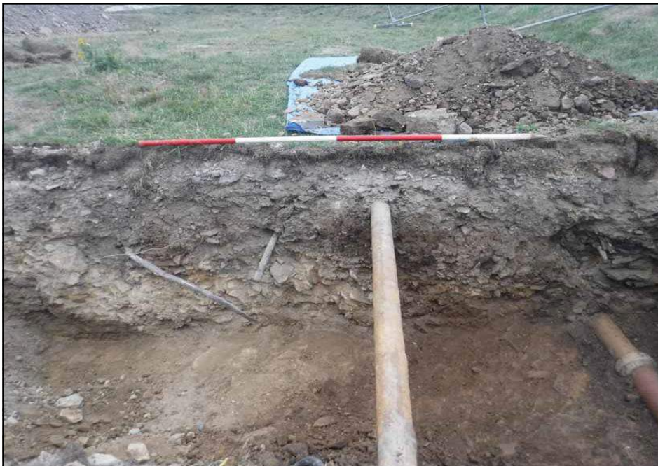
Plate 12. Services in section in Trench 2, looking southwest
