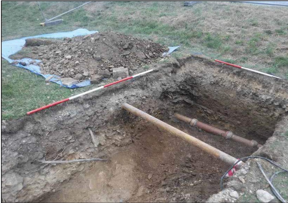
Plate 13. Service pipes in Trench 2, looking northwest
