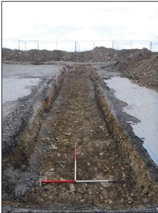
Plate 26. Post-excavation view along Trench 3, looking northwest
