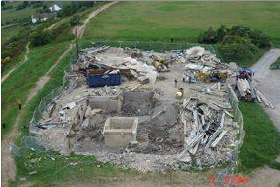
Fig. 4. The site of the hotel at the end of demolition, 2005
