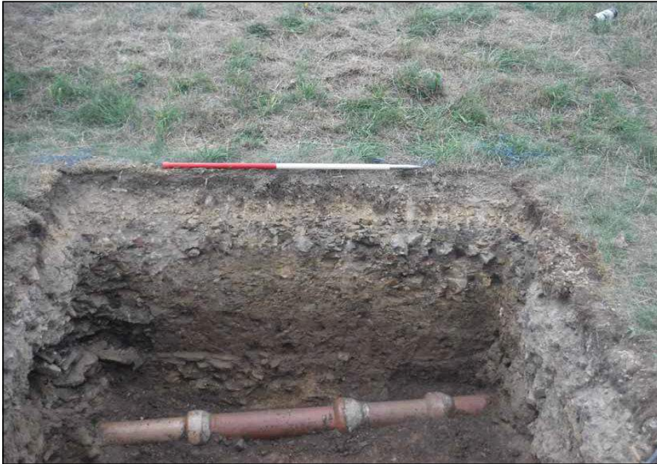
Plate 19. Lower level pipe at northwest end of Trench 2, looking northwest
