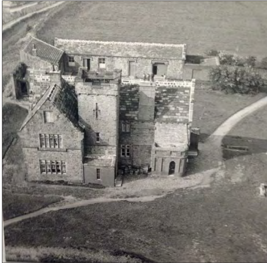
Fig. 4. Photograph of hotel and outbuildings by W.H. Sykes, 1912
