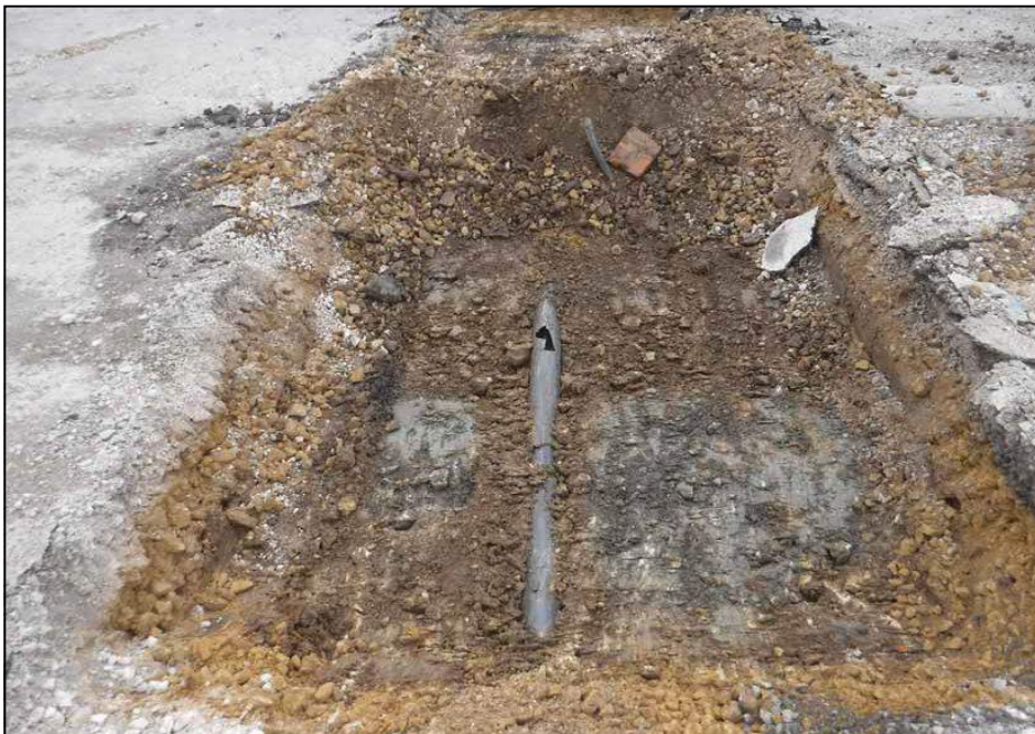
Plate 4. Plastic duct containing services 005 in Trench 1, looking southwest
