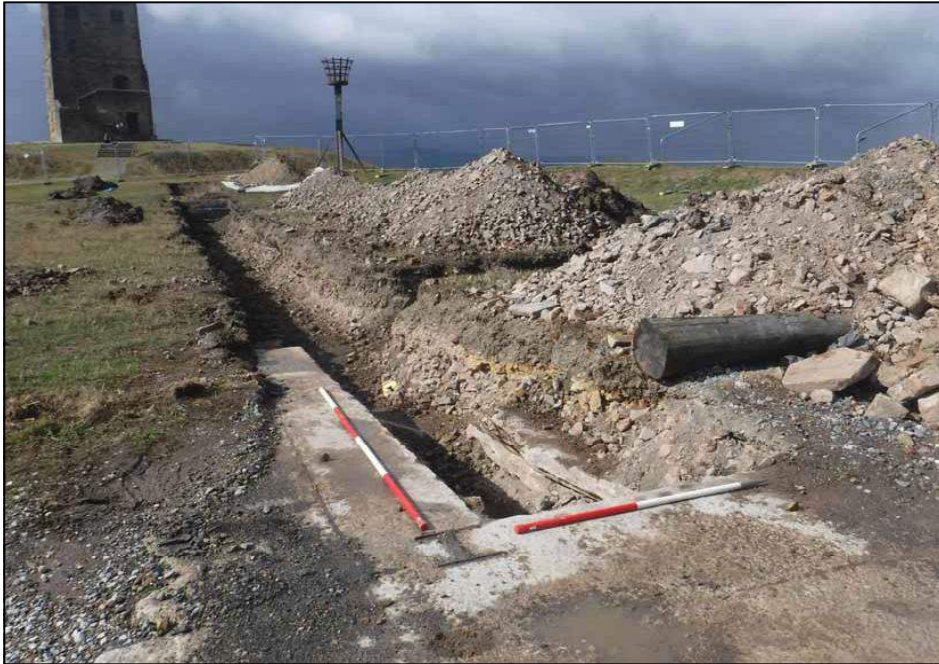
Plate 7. Concrete base for cellar superstructure in Trench 1, looking northwest
