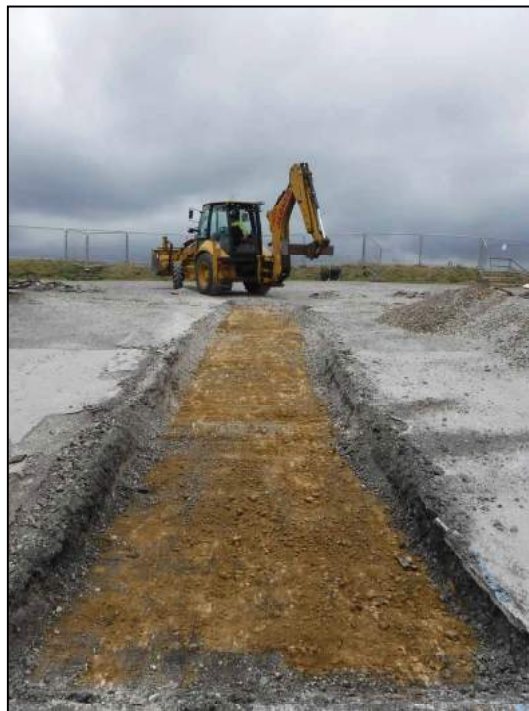
Plate 22. Sandy levelling material under tarmac in Trench 3, looking northwest
