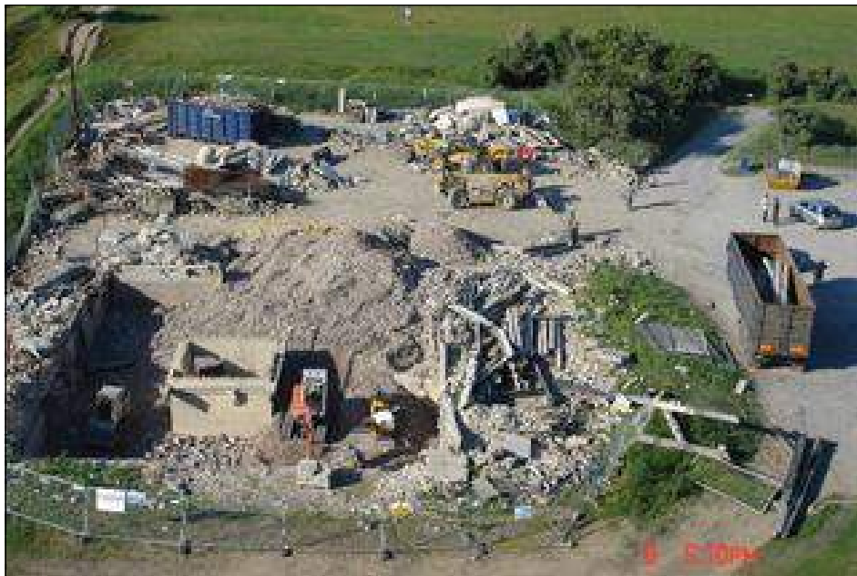
Fig. 5. Filling the cellar with crushed rubble and consolidating the fill, 2005
