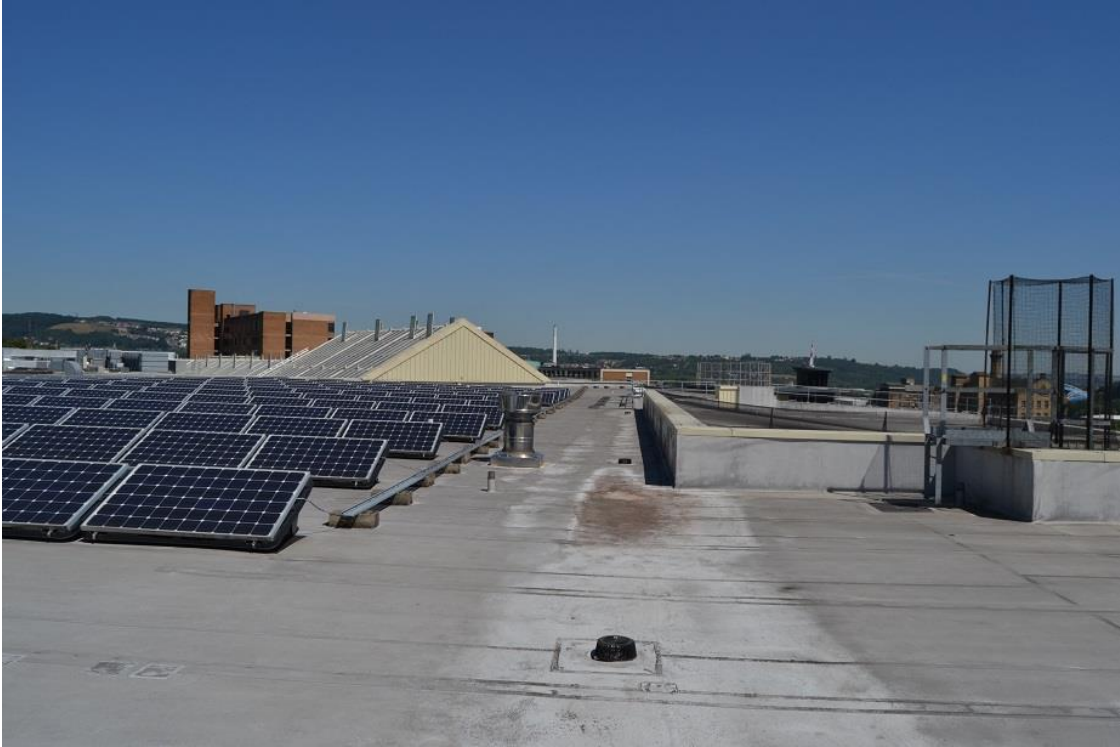
Photo 5 – Roof, as existing
