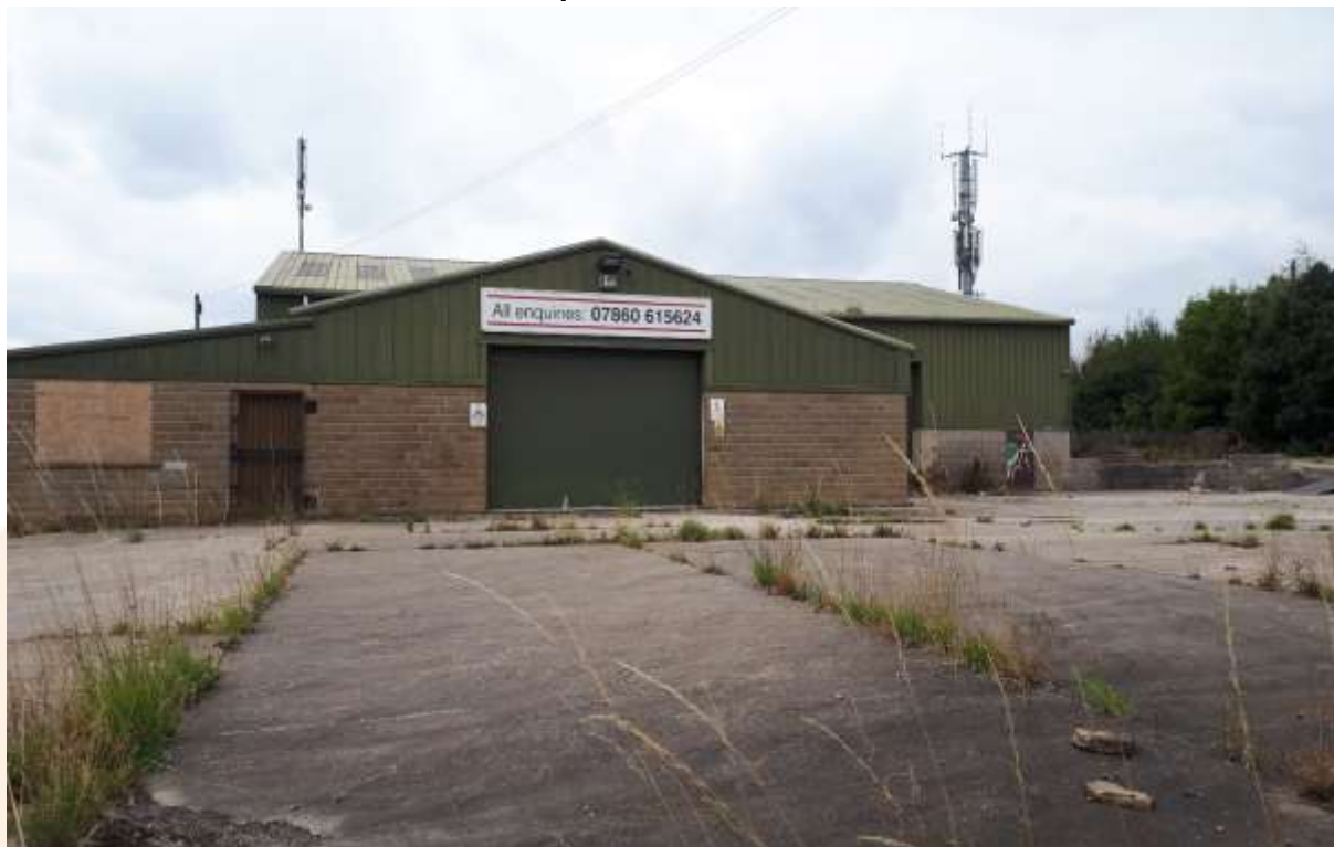
Photo 1: Front of site. North-east aspect
