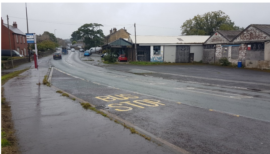
Photograph 2 – Westwards along the A640 New Hey Road
