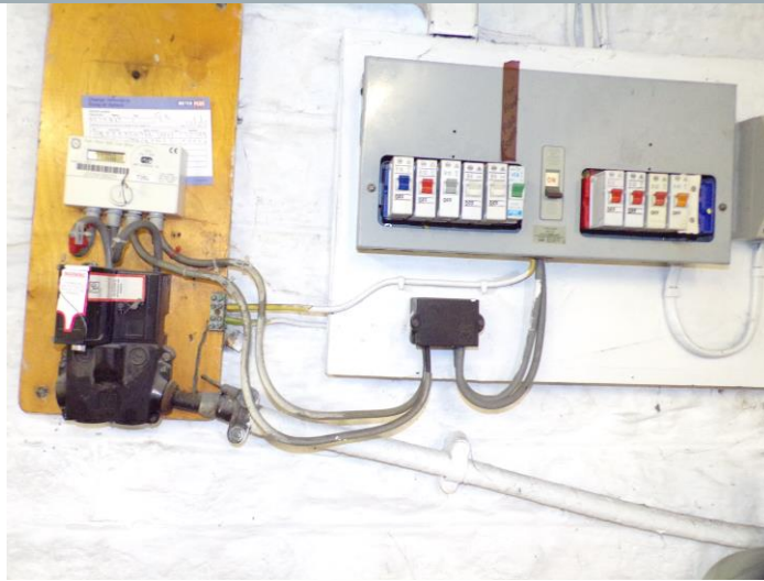
Electric meter and consumer unit
