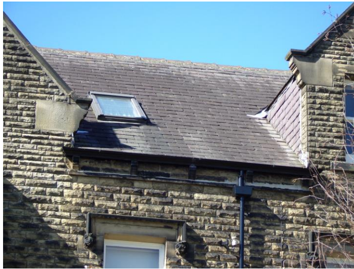
Front roof slope
