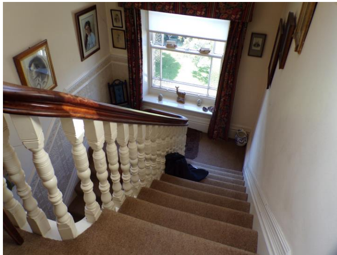
Glazing to stairwell window
