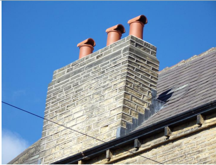
Chimney stack A
