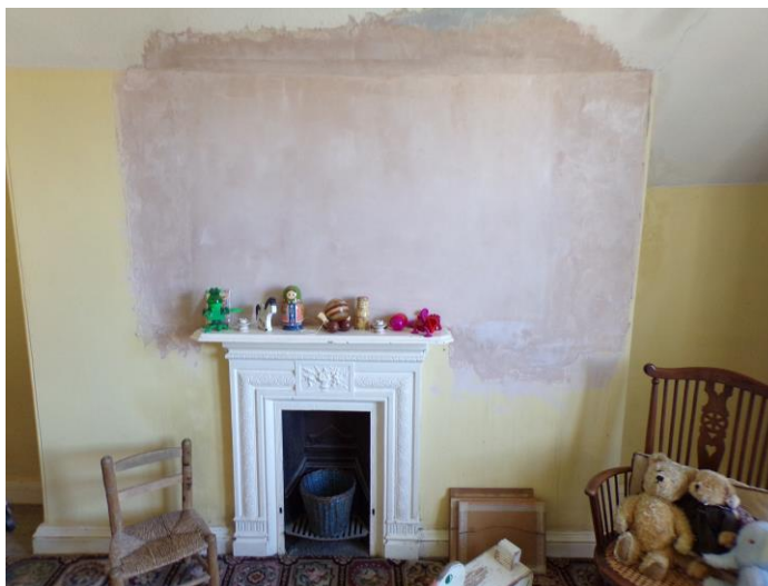
Previous wall repairs
