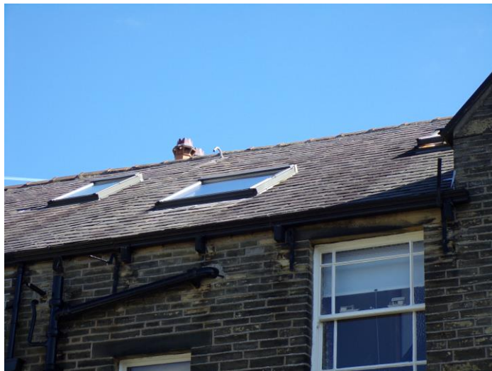
Rear roof slope
