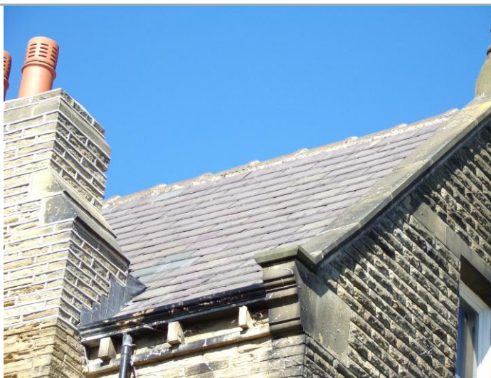
Side roof slope
