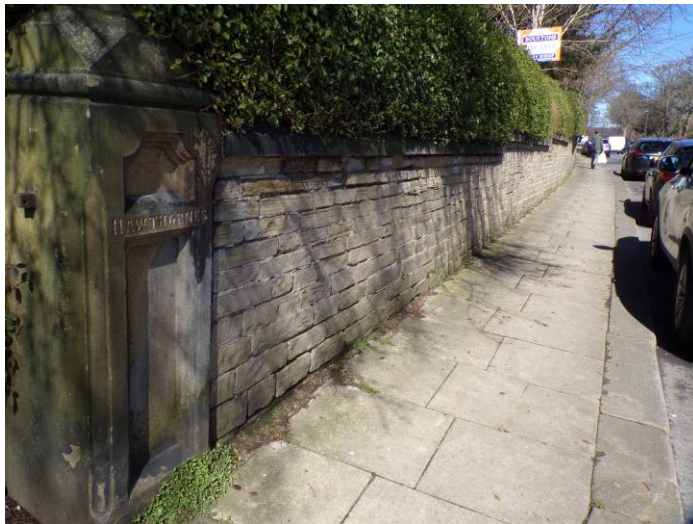
Stone boundary wall
