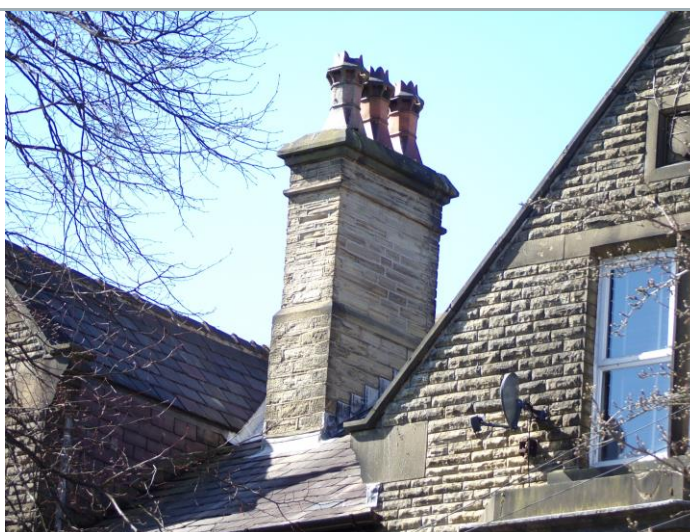
Central chimney stack
