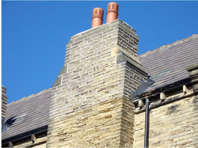
Chimney stack B
