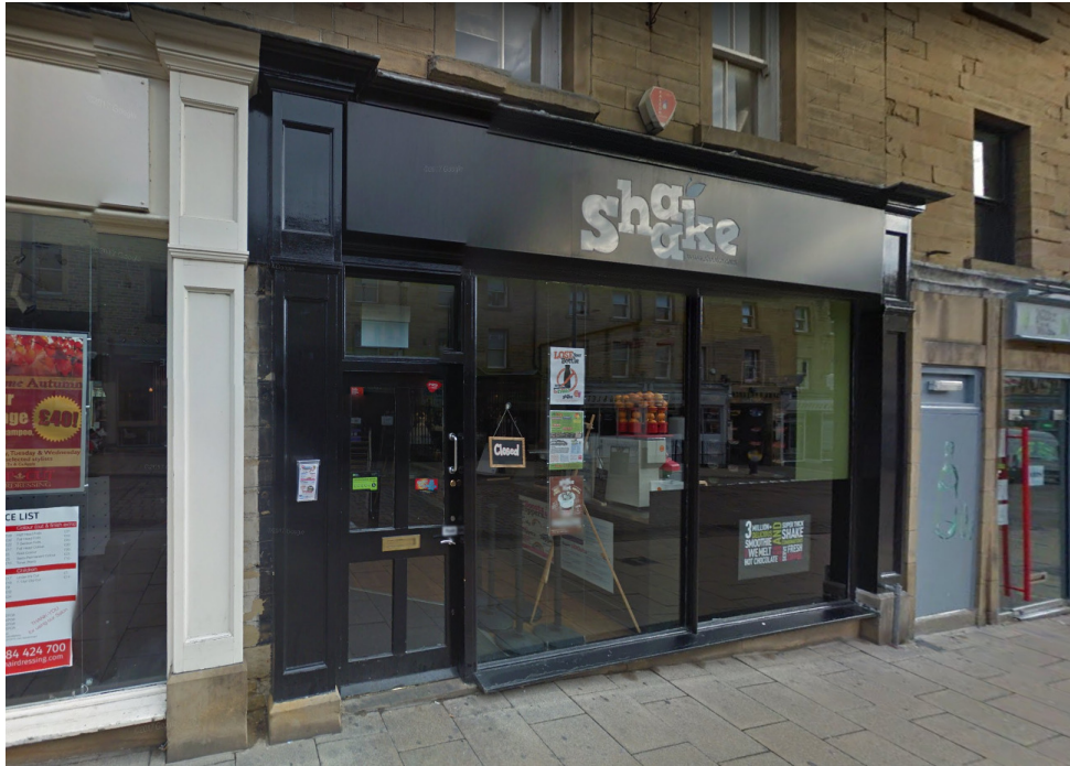
Existing Shop 51 King Street, Huddersfield
