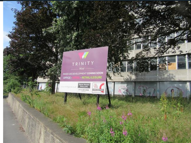
Trinity West scheme hoarding up
