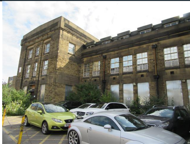
Existing building on site
