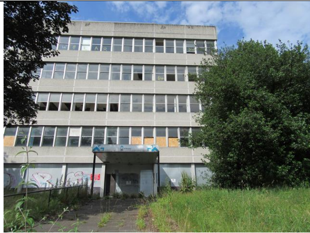
Office building in poor condition on site
