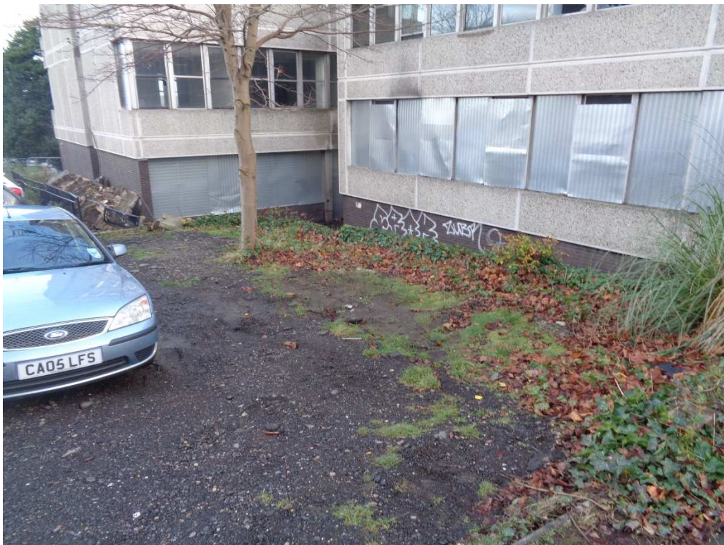
Photograph 6 Elevation changes in the central section of the site.
