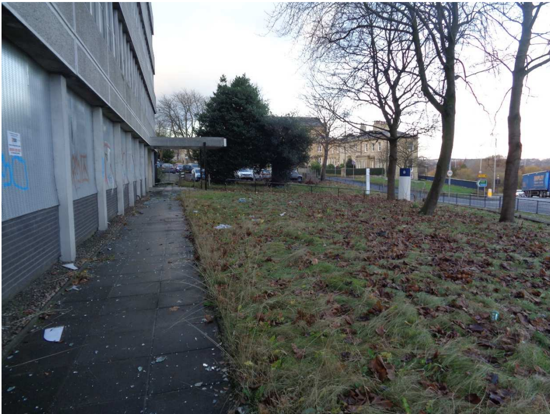
Photograph 8 South-eastern section of the site looking north along eastern boundary.
