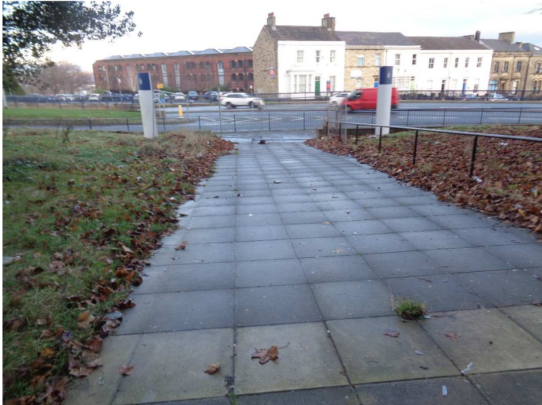
Photograph 7 View south-east towards the junction of Castlegate and Trinity Street.
