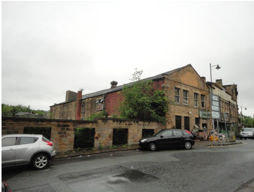
View front Station Road
