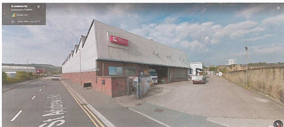
Existing view south along St. Andrew's Road
