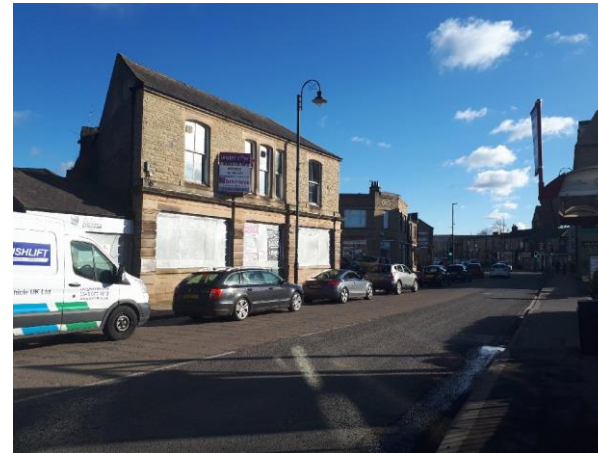
Image 1 – Leading elevation fronting Huddersfield Rd
