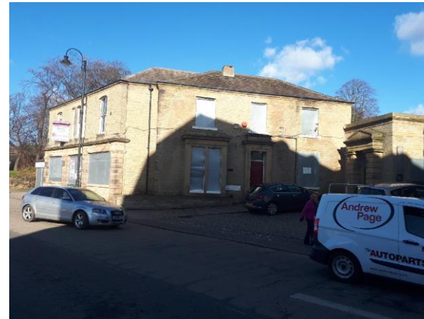
Image 2 – Secondary elevation off Huddersfield Rd
