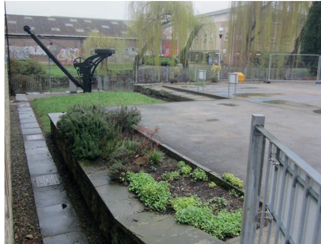
View of transition between Listed building and car park
