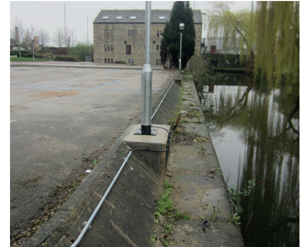
View of existing retaining pavior along canal
