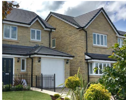
Integral garage with pitched roof
