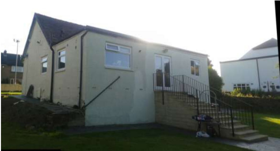
Photo of existing property from rear
