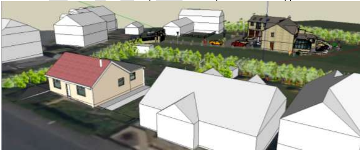
Aerial view of existing
