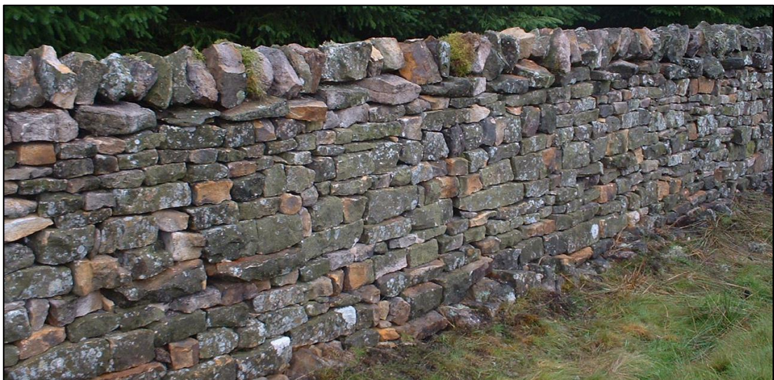
Plate 2. Example of dry-stone wall to protect against encroachment
