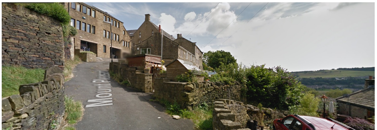
Street view – west elevation of 1 Mount Pleasant, looking north east.
