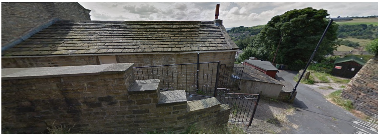
Street view - rear of 1 Mount Pleasant, looking south west.
