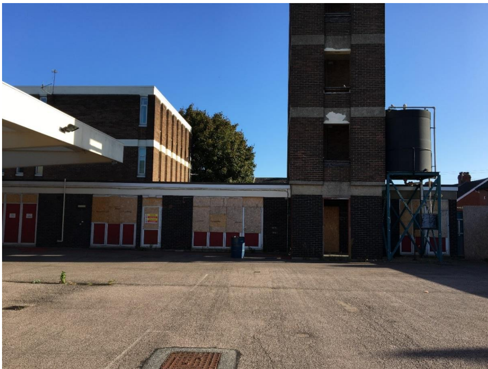
Figure 3: Offices with ancillary accommodation and training tower attached to 3-storey administration block
