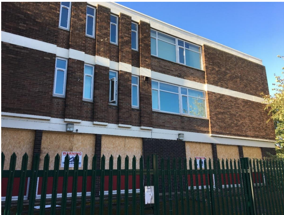
Figure 5: 3-storey administration block as viewed from un-named connecting road
