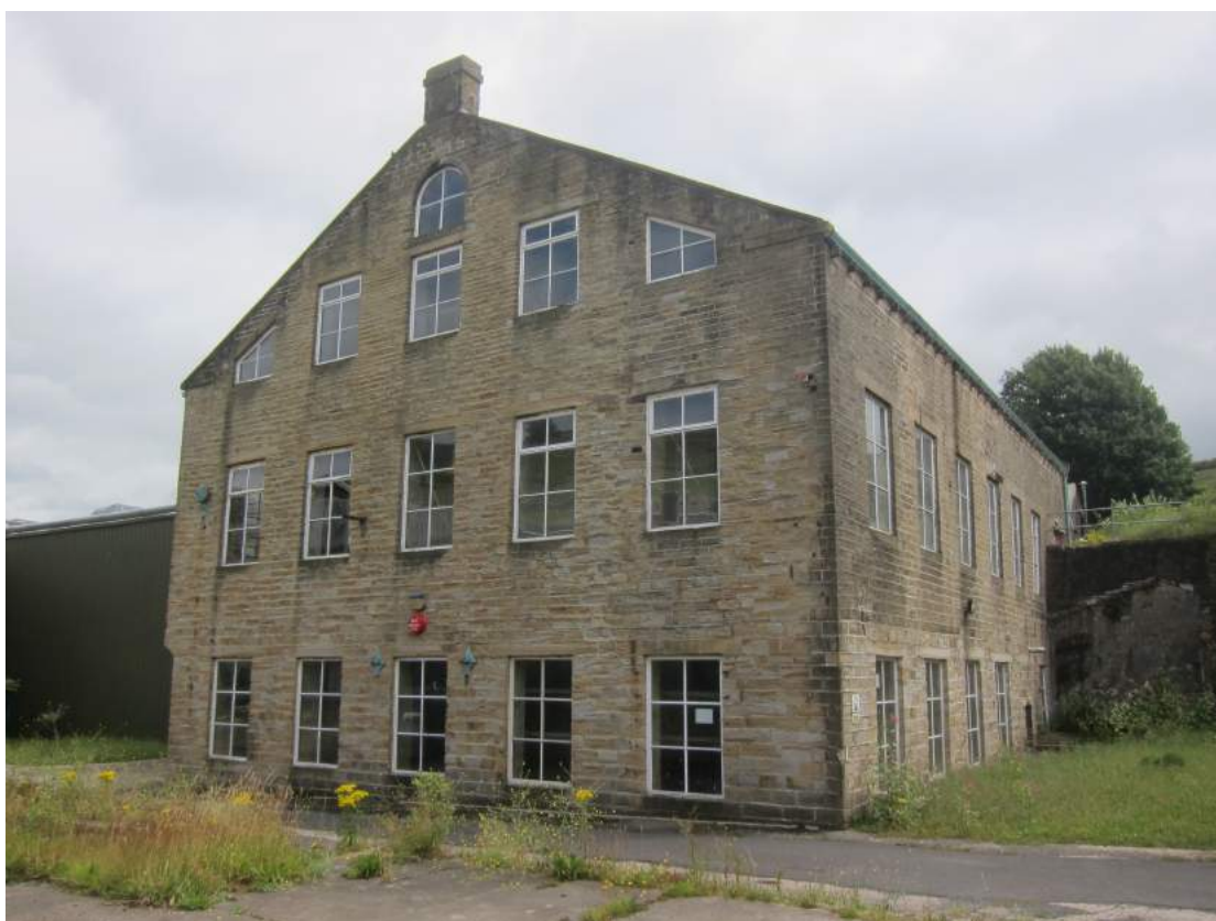
. Figure 5: Mill as existing 1
