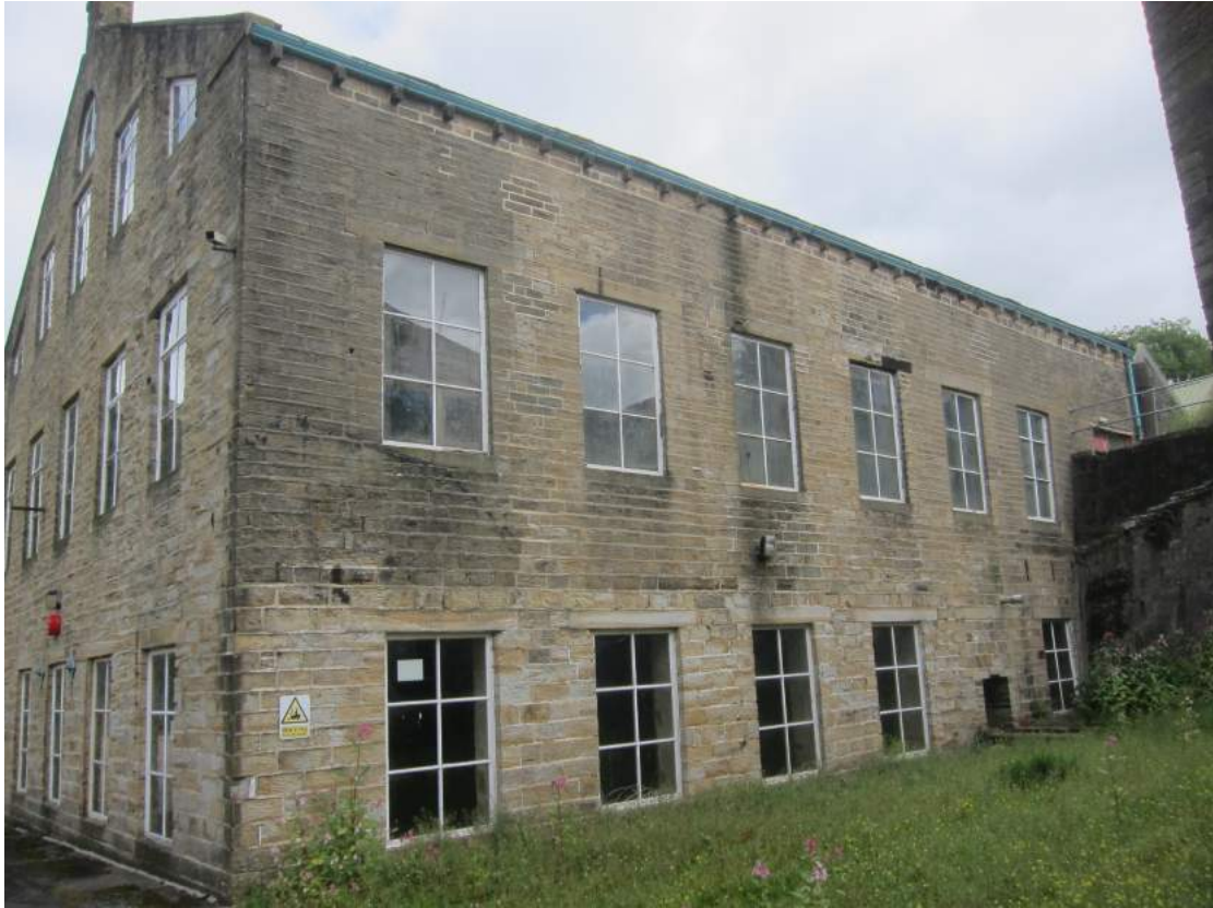
Figure 6: Mill as existing 2
