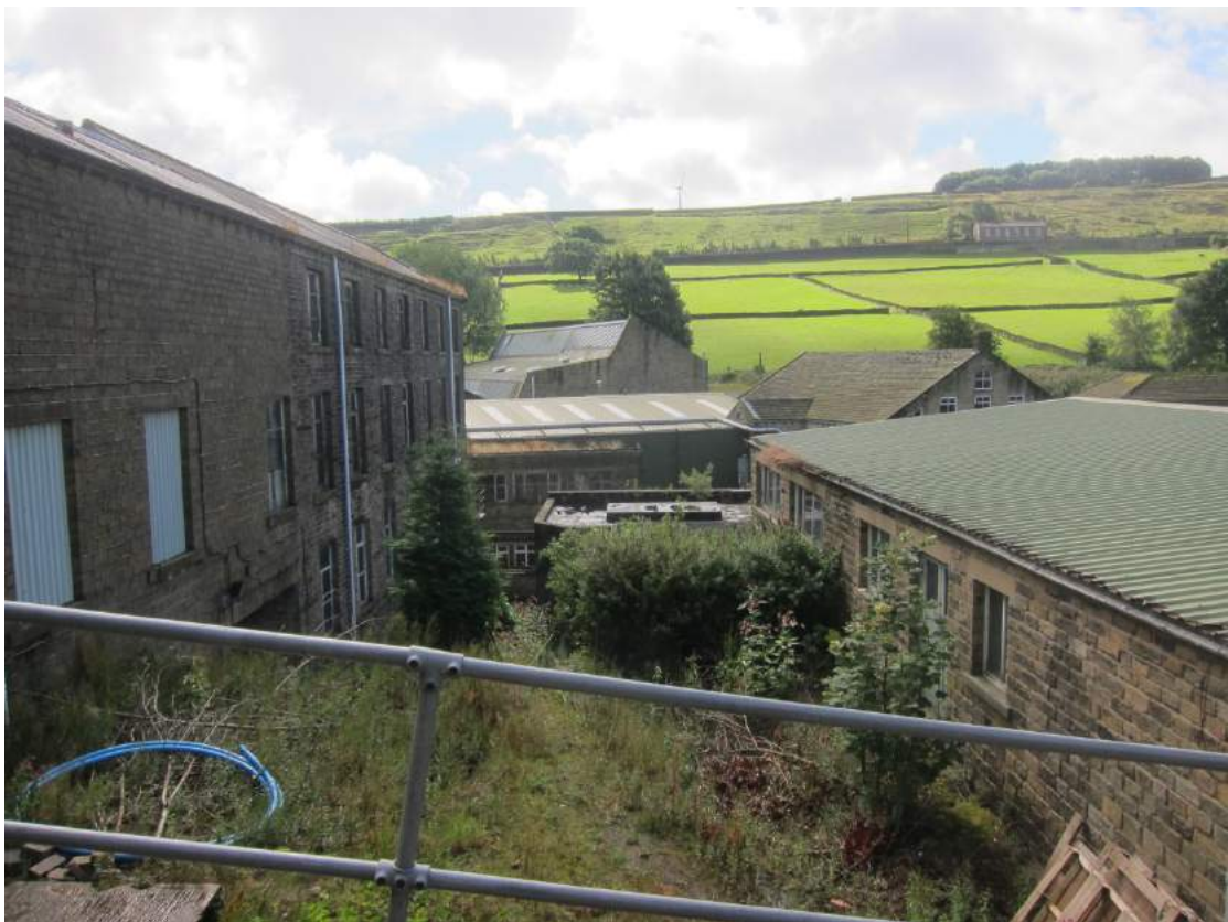
Figure 9: General view of haphazard site development with gable of listed building at rear right plus curtilage listed buildings with beautiful countryside beyond
