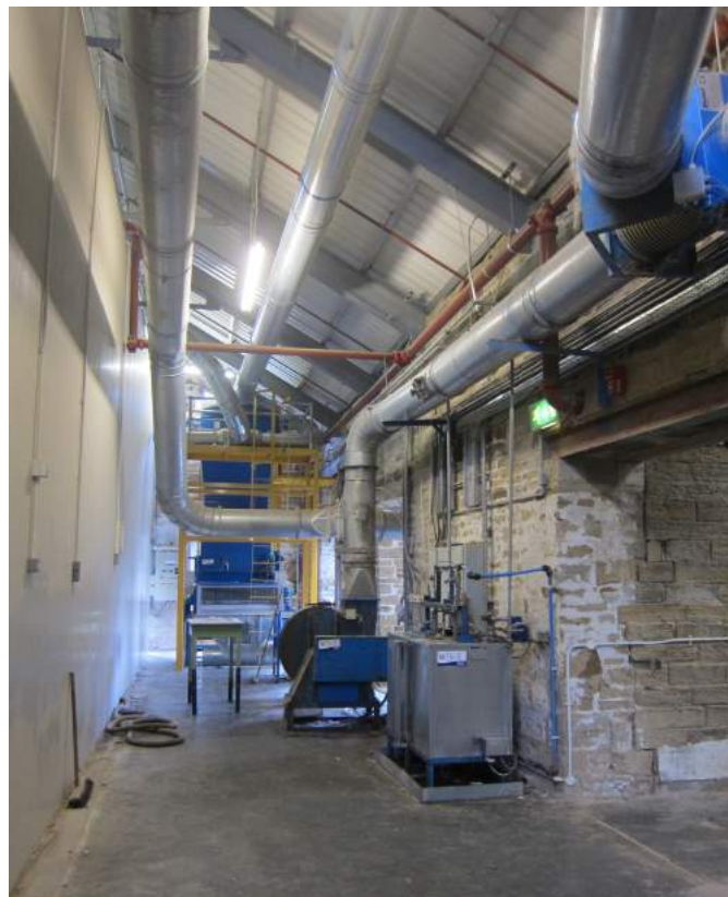
Figure 4: Machinery installed on the upper floor. The replaced roof structure can be seen.
