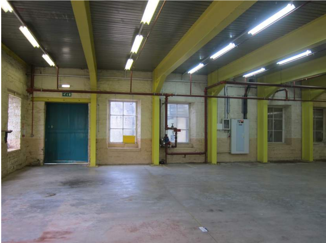
Figure 3: Original internal structure removed and new steel frame inserted
