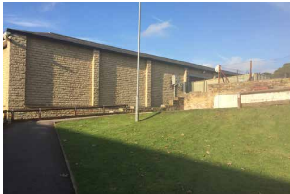
View of the pedestrian connection and adjoining Co-Op boundary
