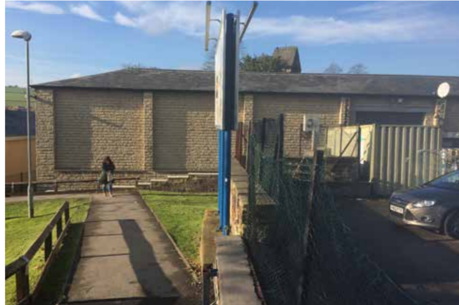
View of the existing pedestrian connection from the site
