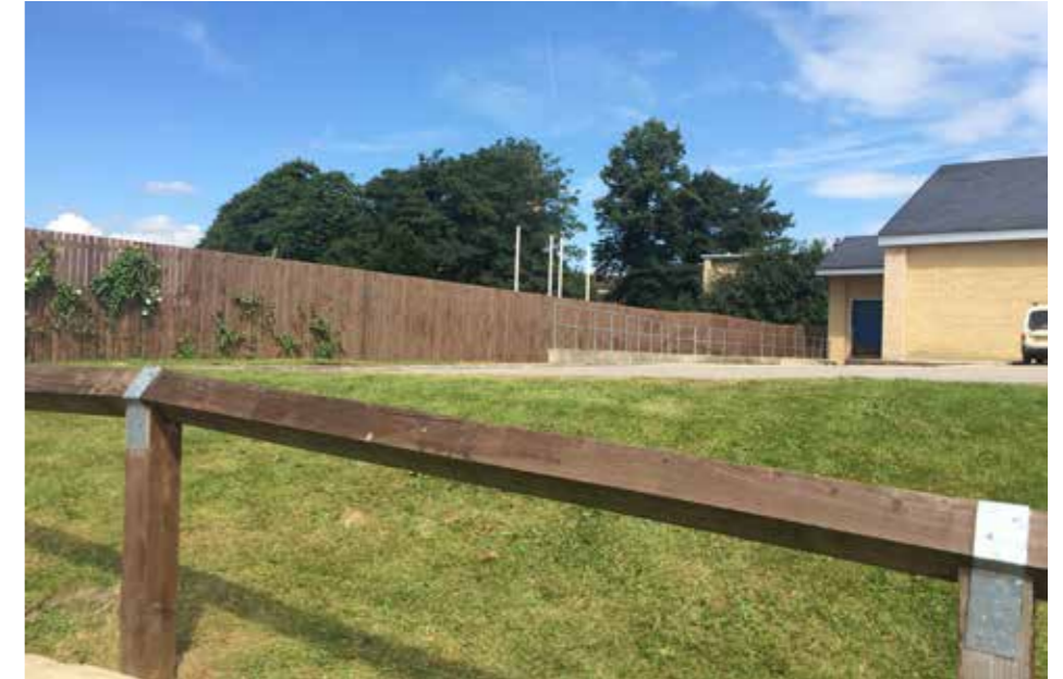
View of the boundary with the adjoining Newgate site which is currently under construction
