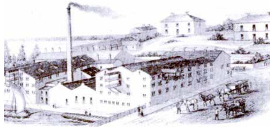
EAST THORPE & RAVENSTHORPE MALT HOUSES
