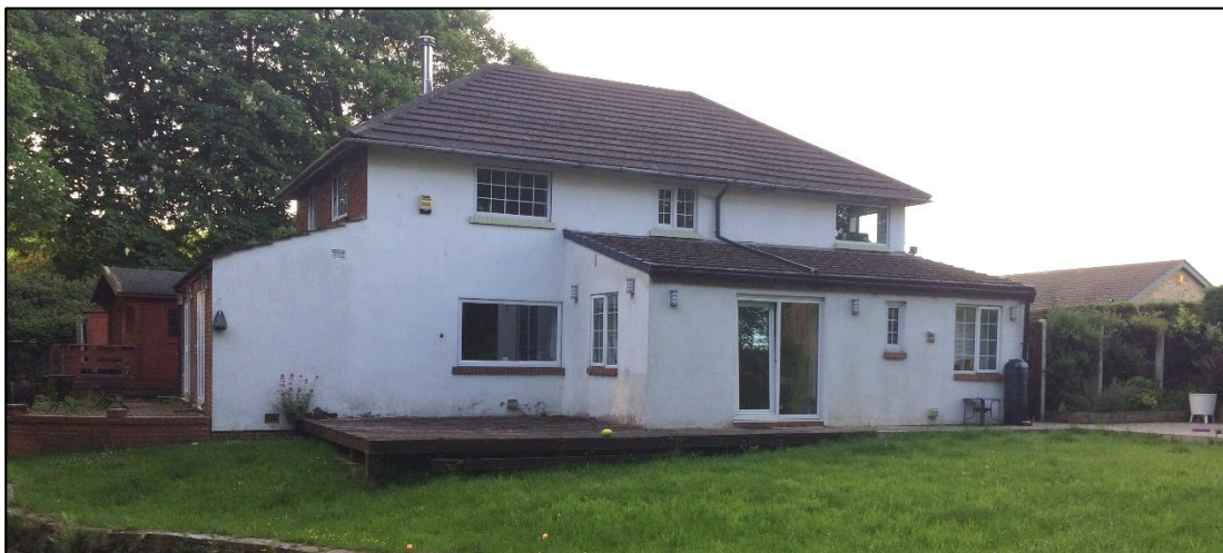
Plate 2. The south elevation of the surveyed building
