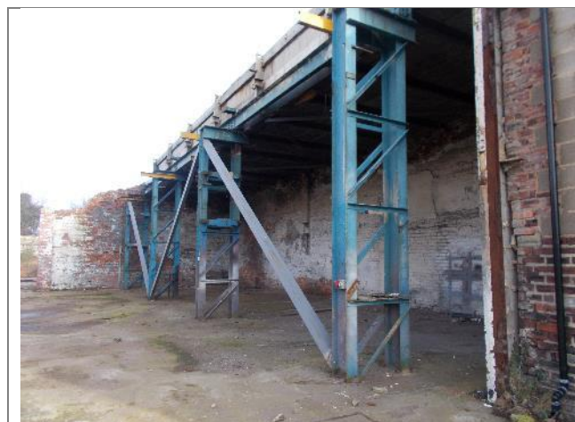
Plate 3: Open fronted building supported by metal frame.
