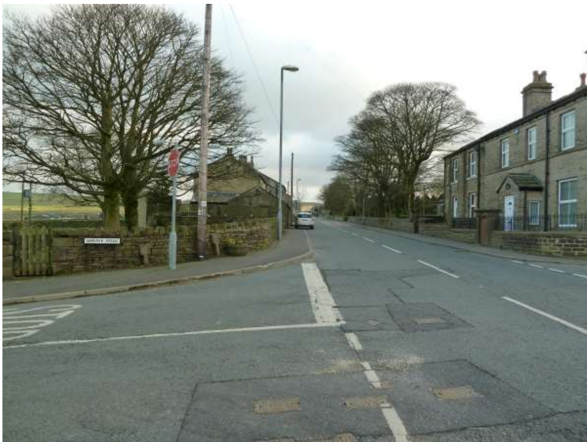
Greave Road junction with Dunford Road looking south
