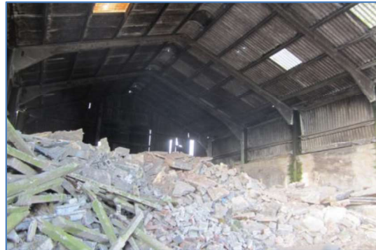
Photo 2 - Interior to building 1.
