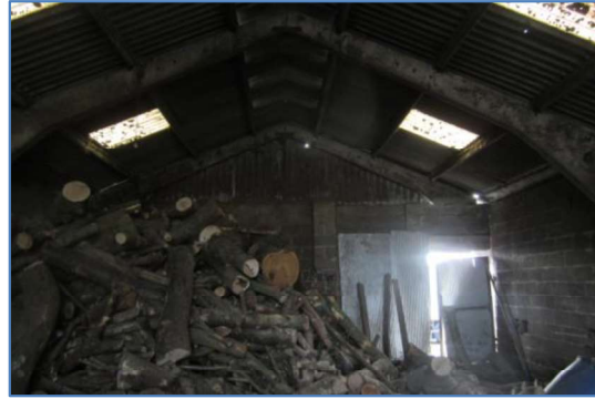
Photo 26 - Interior to building 12.
