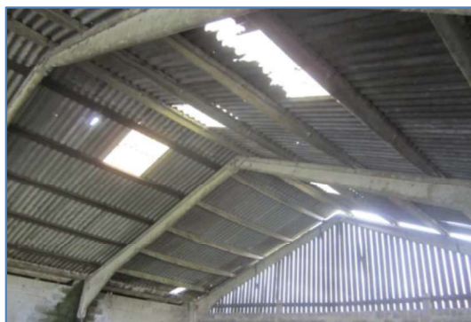
Photo 16 – Interior of building 7.
