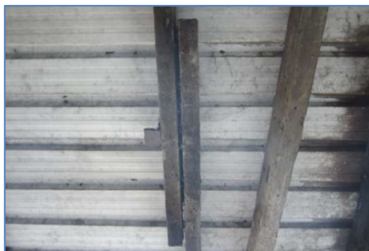
Photo 14 – Overlapping timbers of building 6 with gaps in-between (cobwebby).
