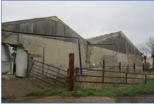
Photo 25 - Rear (south) elevation of buildings 11 and 12.
