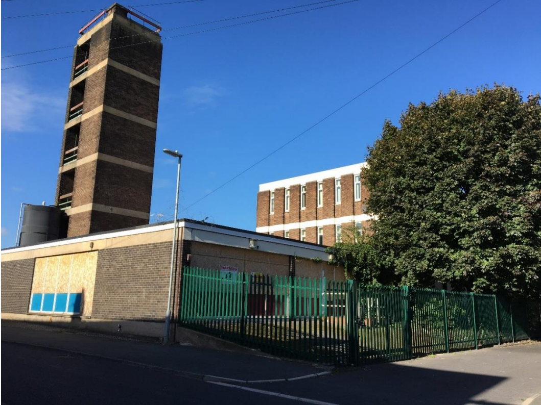
Figure 8: Offices with ancillary accommodation and training tower attached to 3-storey administration block as seen from corner of Broad Street and un-named connecting road
