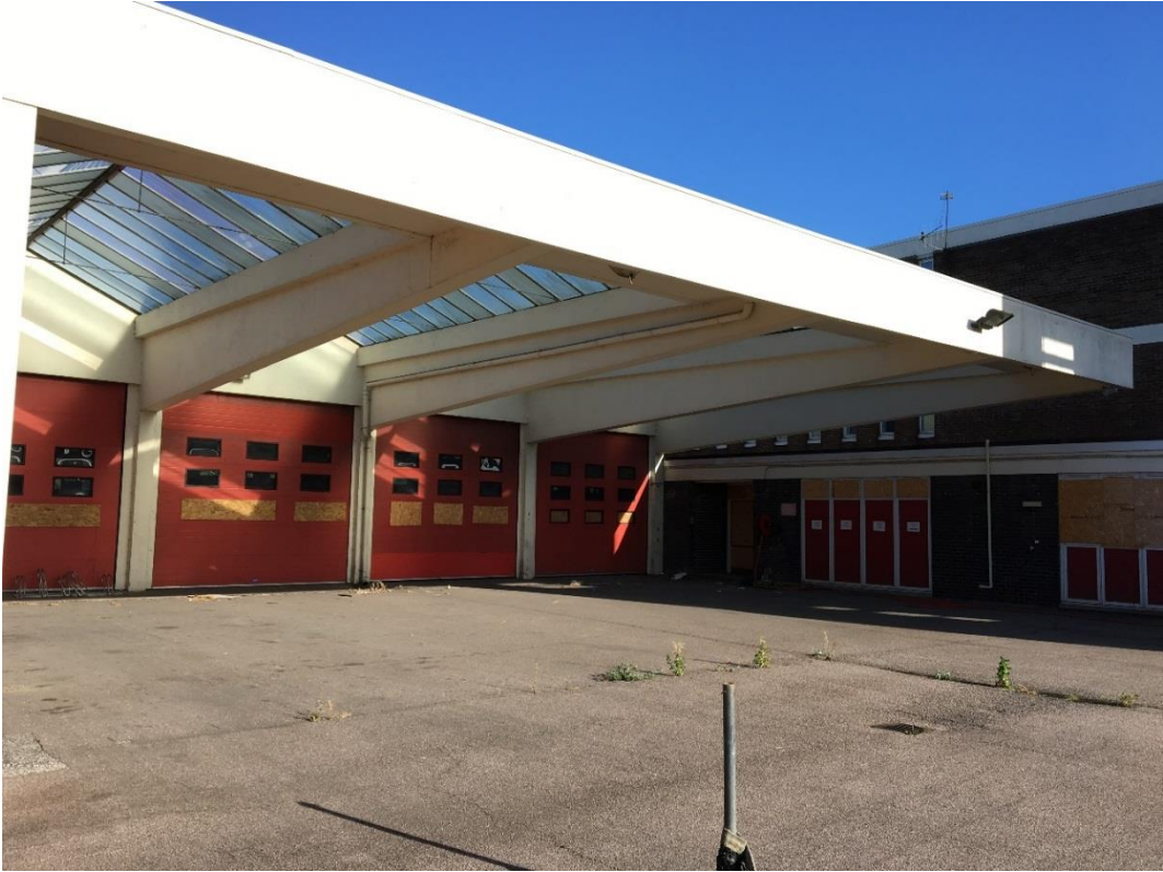
Figure 5: Rear of fire appliance bays with glazed canopy
