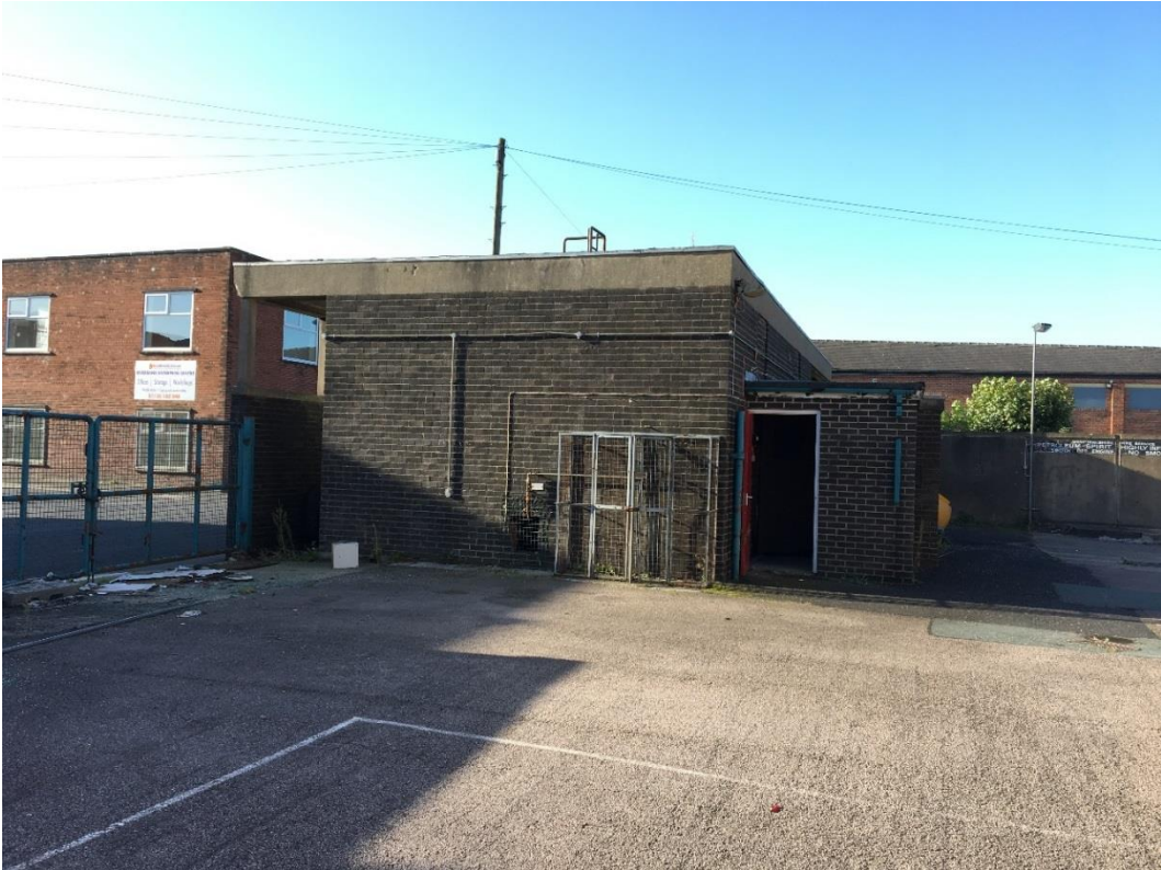
Figure 7: Detached smoke room to South of site
