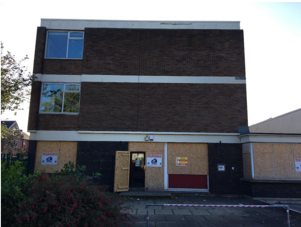
Figure 1: 3-storey administration block as seen from Huddersfield Road
