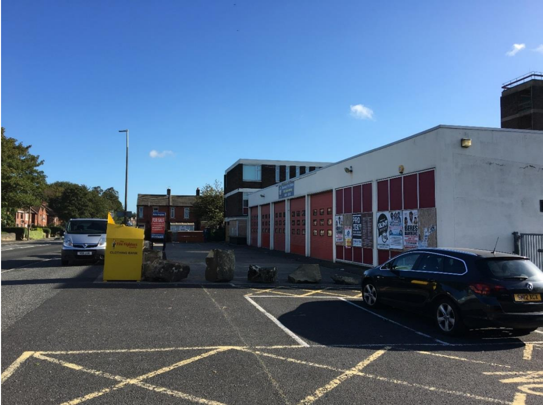
Figure 2: View of existing fire station as seen from Huddersfield Road
