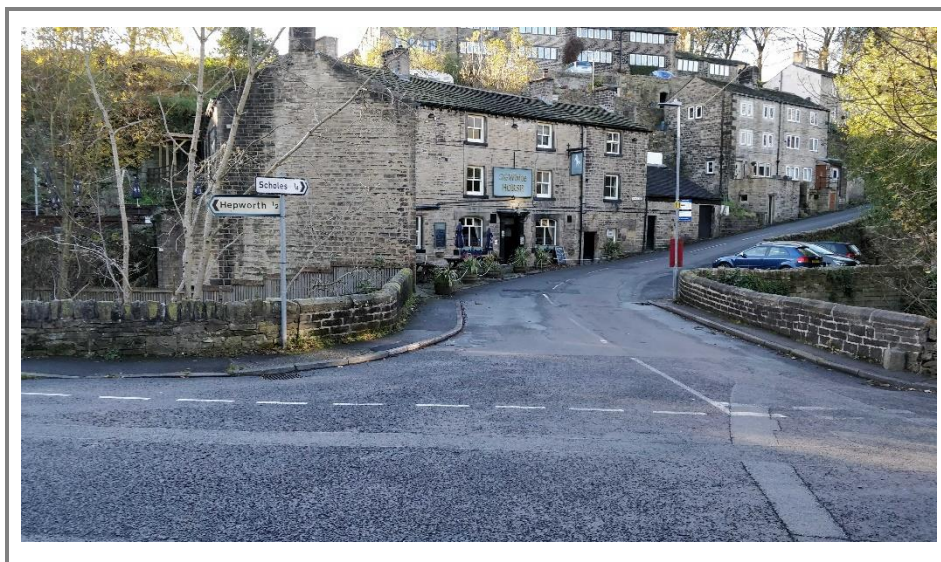
Photograph 3 - View of footway provision on Scholes Road
