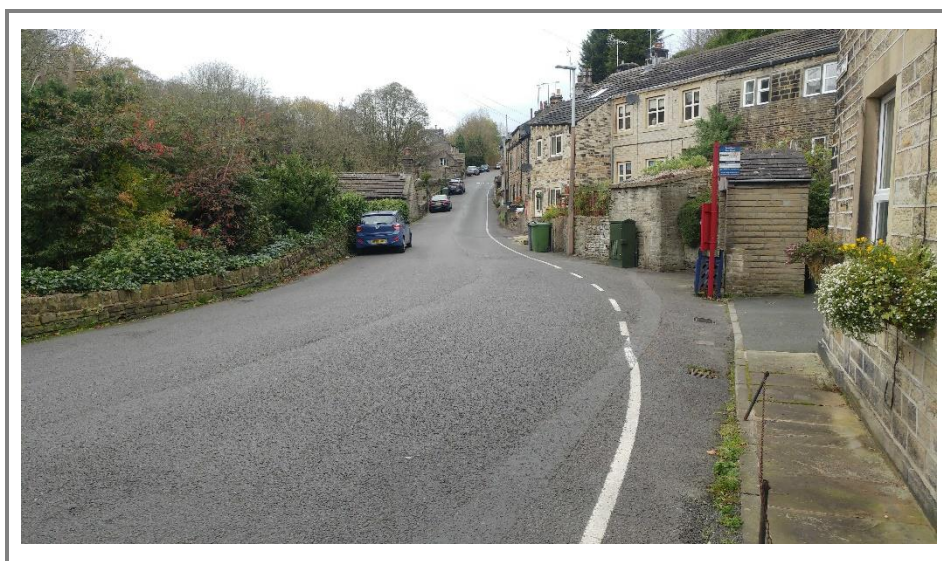
Photograph 7 - View of Bank Street – footway provision on right.
