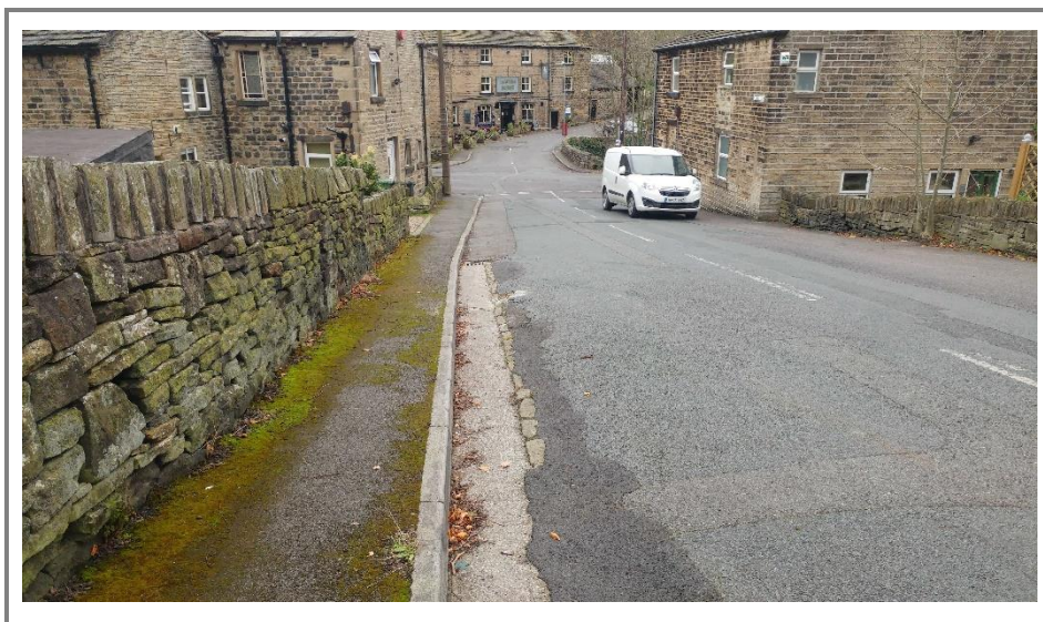
Photograph 4 - View of southern footway on East Street looking towards Hepworth Road junction.
