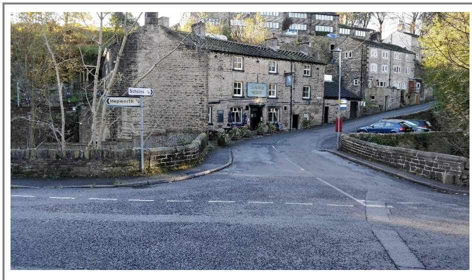
Photograph 3 - View of footway provision on Scholes Road
