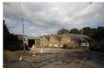
View of mill building from car park
