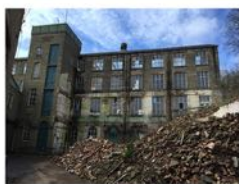
Existing Mill Building to be Retained
