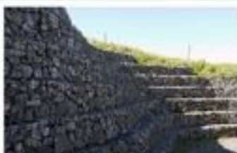
Gabion Basket Retaining Wall
