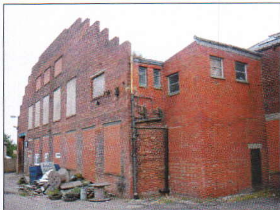
Front of the factory facing north west
