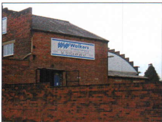
View of factory roof seen from the east
