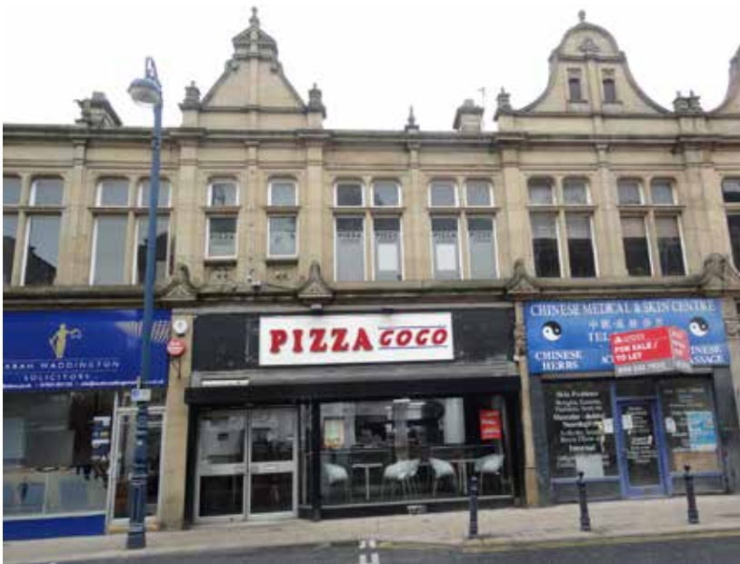
Figure 2 - Existing elevation to Corporation Street
