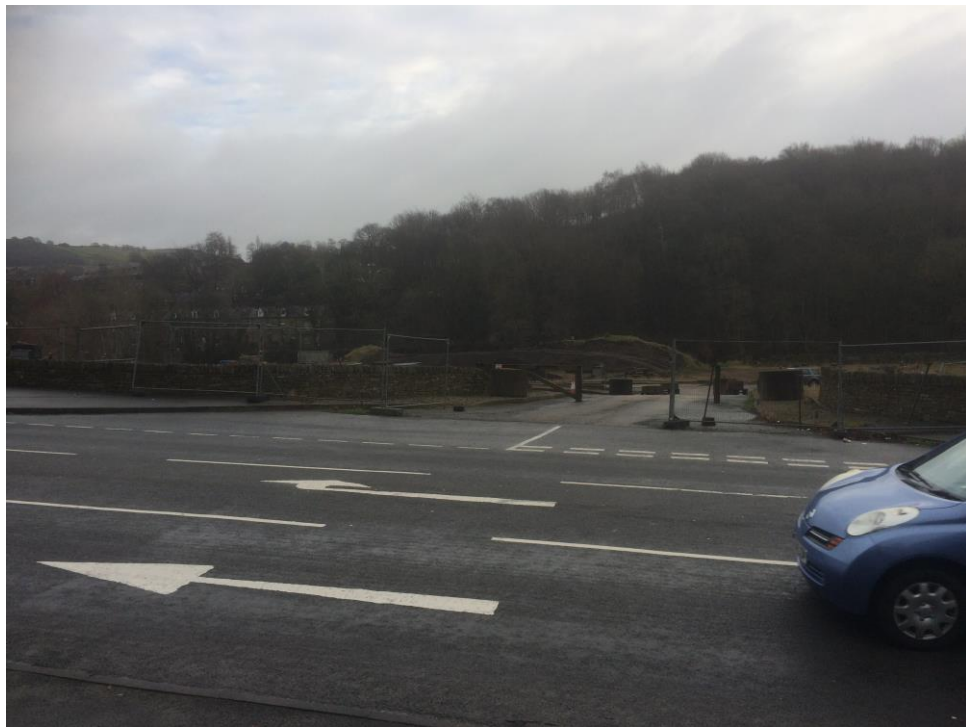
Photograph 2 – Existing Access Road
