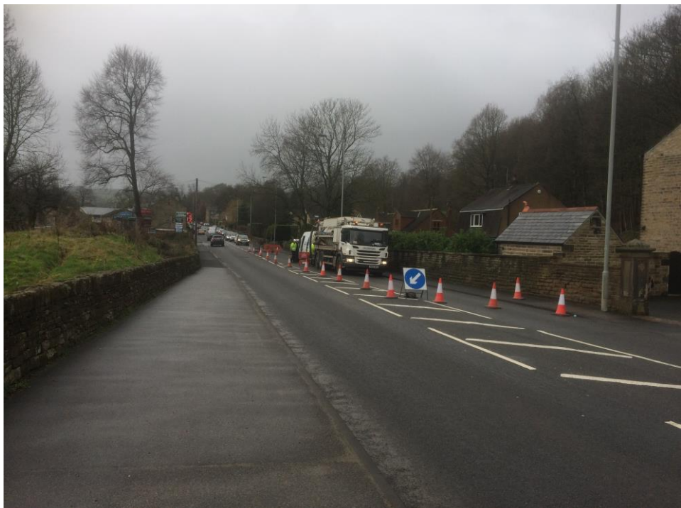
Photograph 4 – Huddersfield Road (to the southwest)
