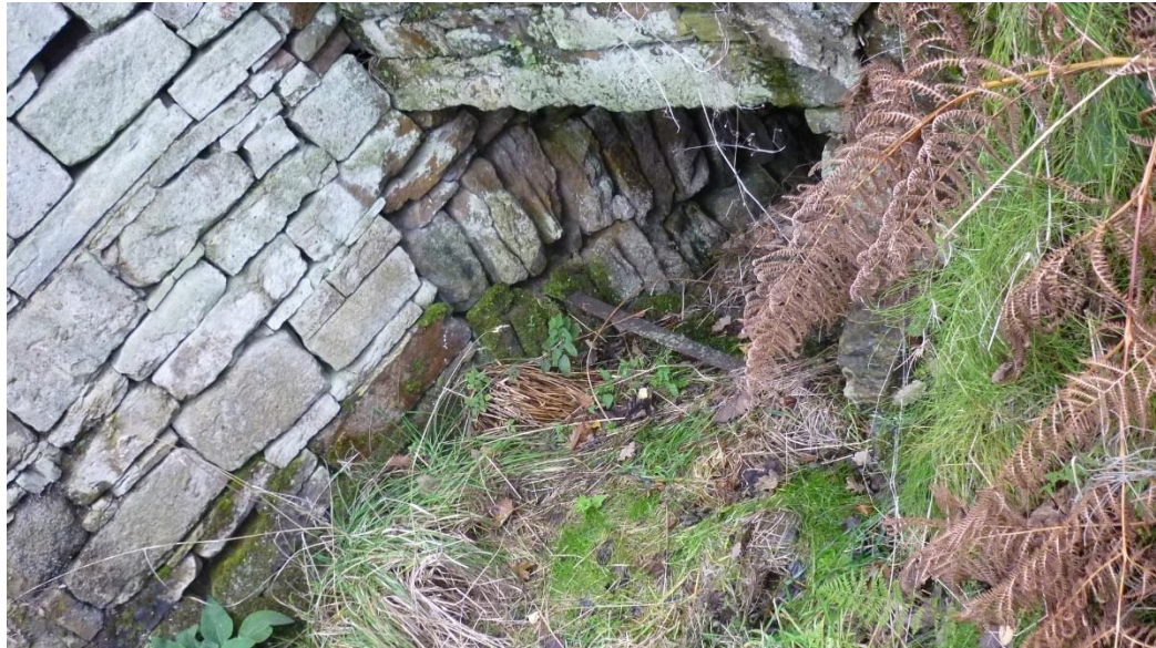
Photo 9: Lower part of the culvert taking dam overflow.
