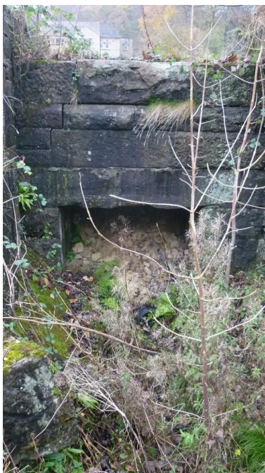
Photo 8: Upper part of the culvert taking excess water from the former dam. Surface water pipe just visible.
