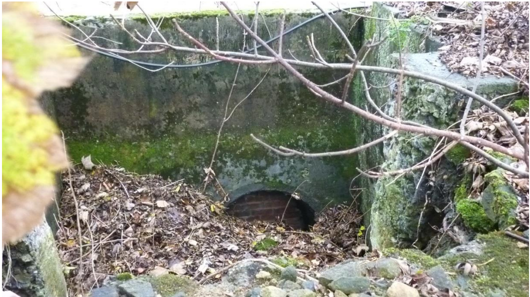
Photo 5: Outlet in the dam wall for the turbine water
