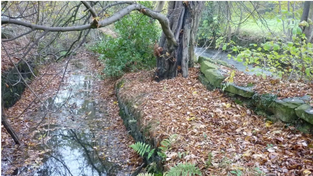
Photo 6: Culvert (to the left) shortly before the confluence with the River Holme (to the right)
