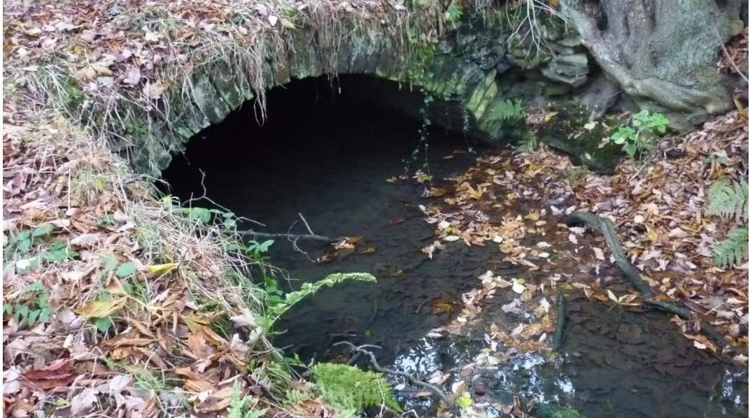
Photo 7: Culvert formerly used for the turbine water
