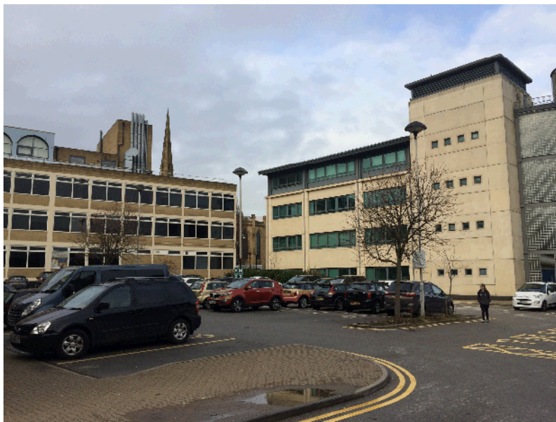
View from Technology building into courtyard – location of link extension
