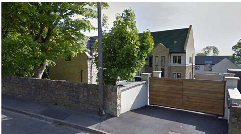
Street view of former no.46
