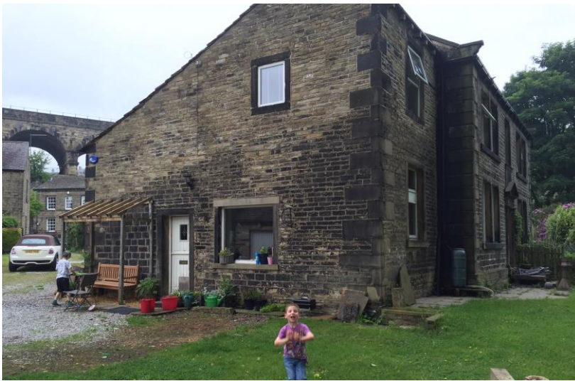
Side elevation of existing house.
