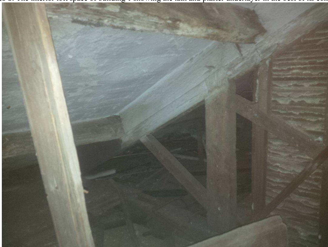
Photo 8: The interior loft space of building 1 showing the lath and plaster underlayer in the best of its condition
