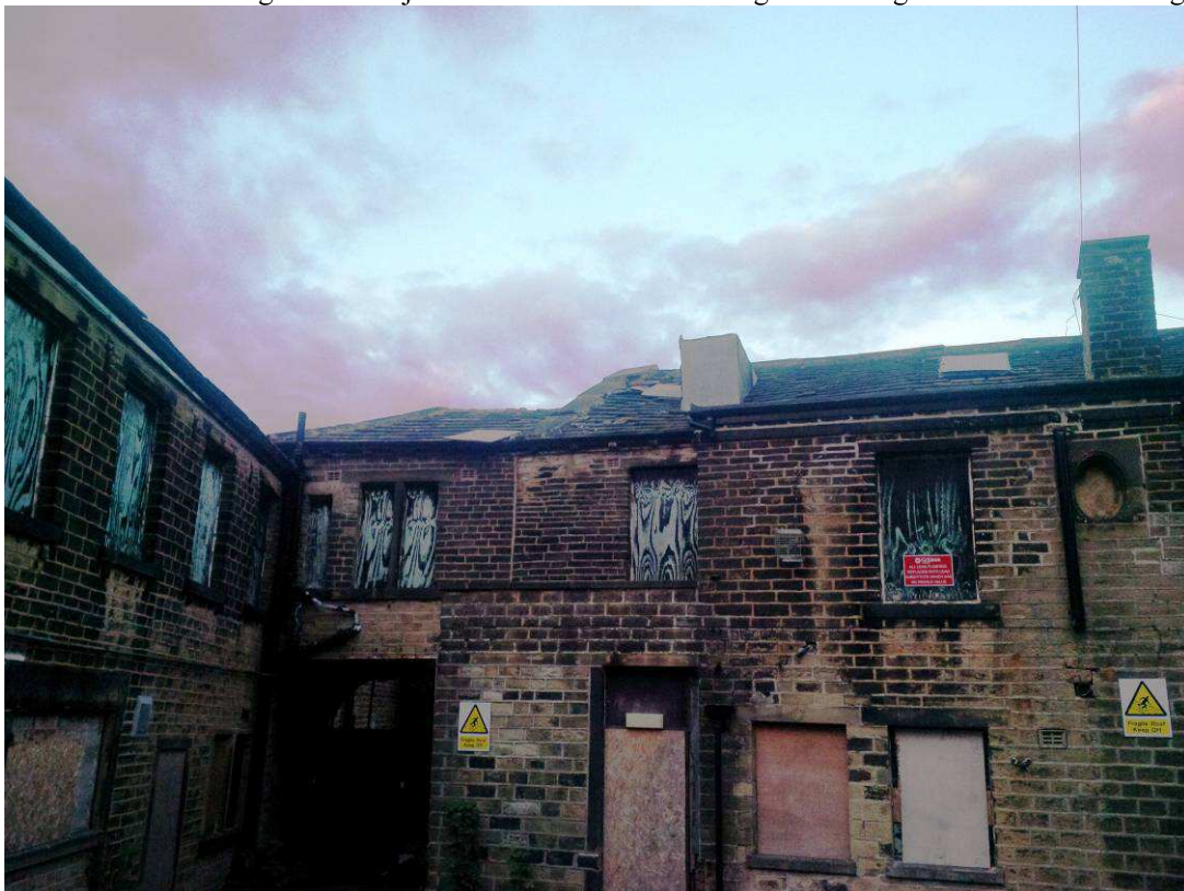
Photo 4: West wall of building 1 where it joins the south wall of building 2 including the 1 st floor connecting corridor
