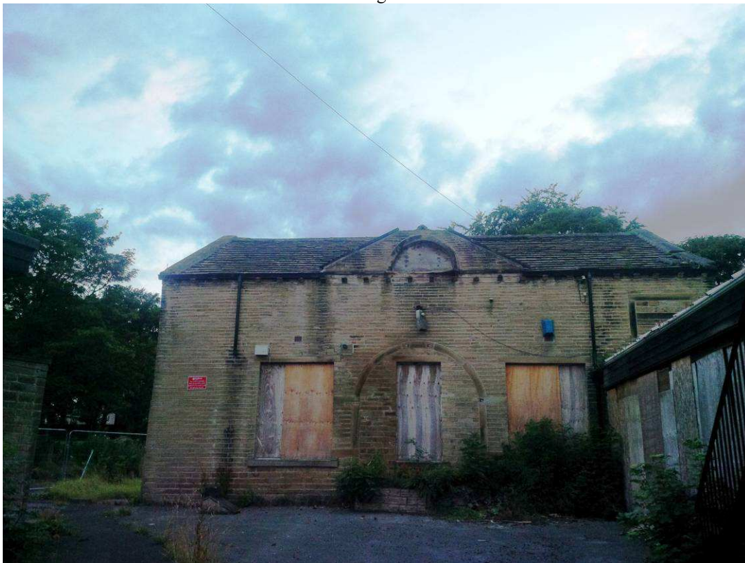
Photo 3: Building 3 from the east
