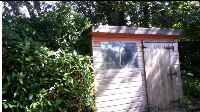
Photo 5: B3 western elevation
