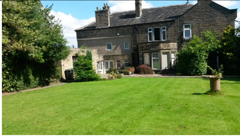
Photo 1: B1 western elevation
