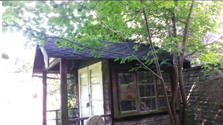
Photo 4: B2 northern elevation
