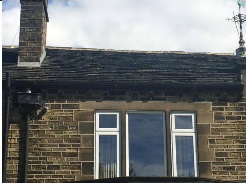
Photo 2: B1 raised tiles western roof pitch
