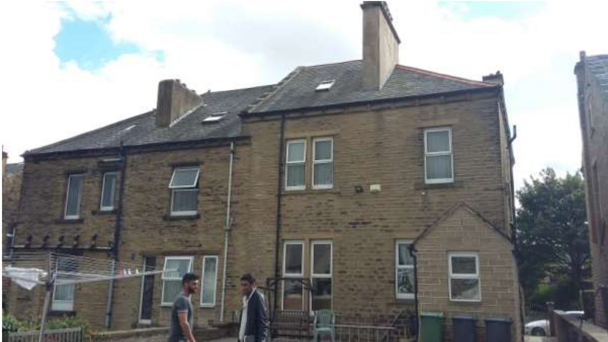
Rear view of existing with very tall chimney
