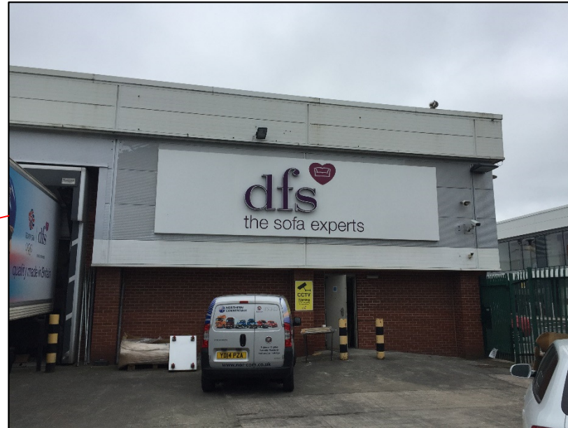
Rear Elevation View (East)
