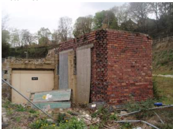
Photo 2 TG4 (retaining wall) at north site boundary
