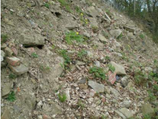
Photo 8 Retaining wall detail
