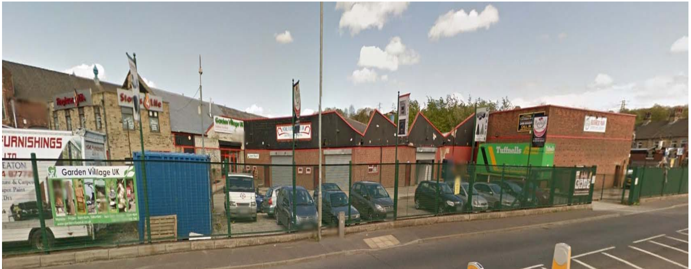
Front view showing location of Proposed show room
