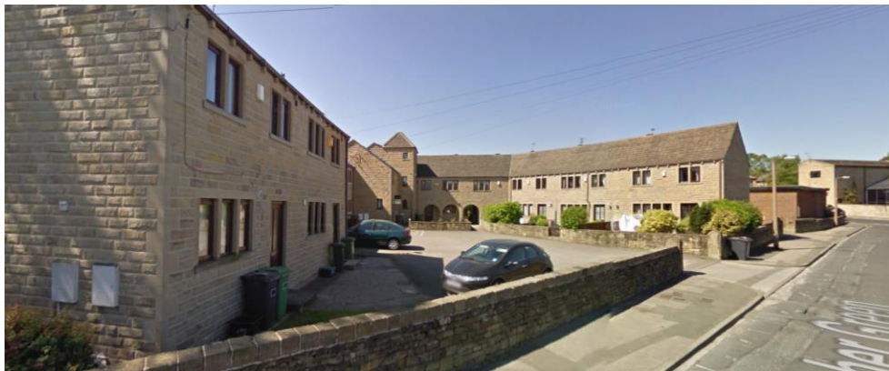
Courtyard Development on Fisher Green
