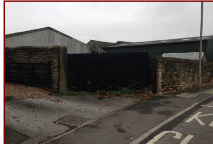
Figure 2.2: A view of the south-western boundary from Barnsley Road
