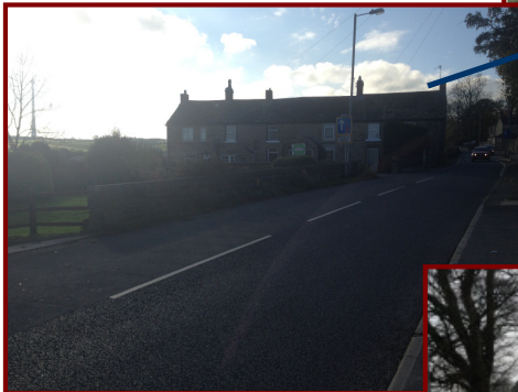
View from site access looking in a westerly direction at nearby cottages at the south side of Barnsley Road
