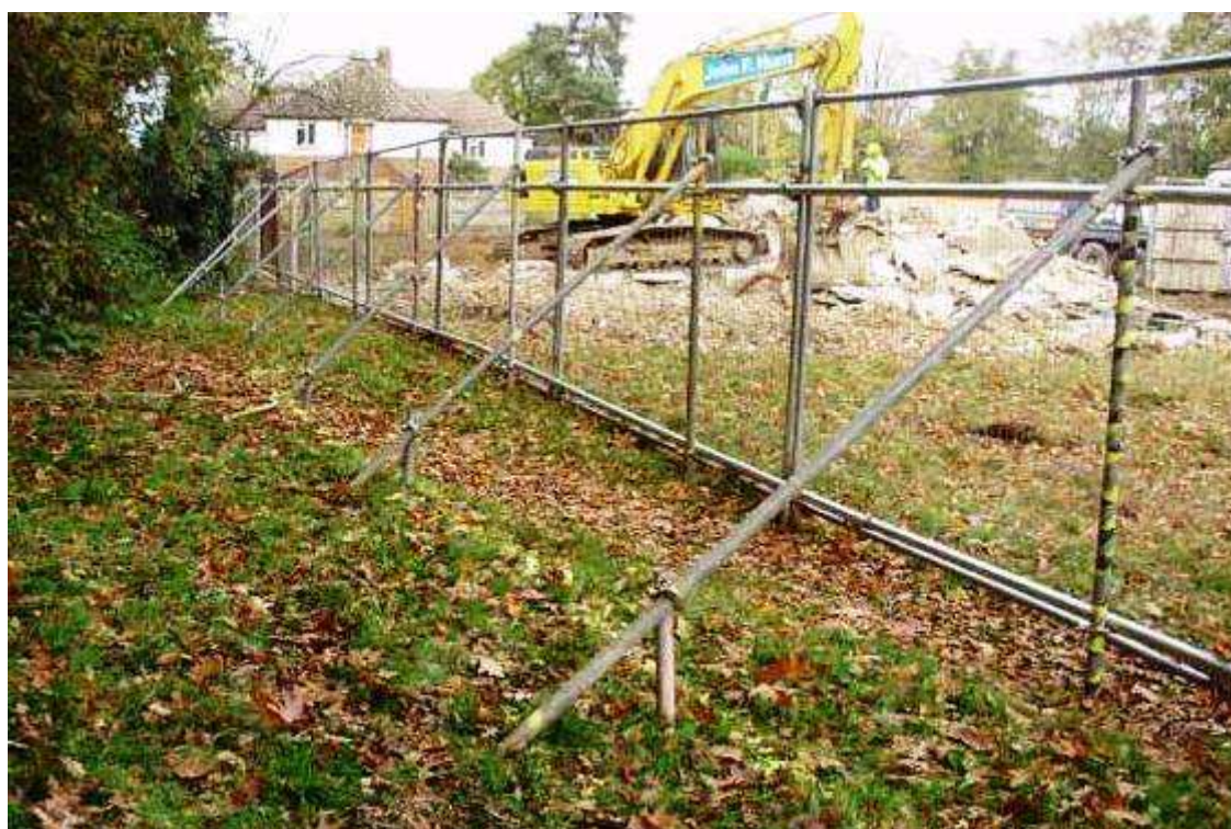
Figure 2: 'Photo of Fencing to BS 5837: 2012'.
