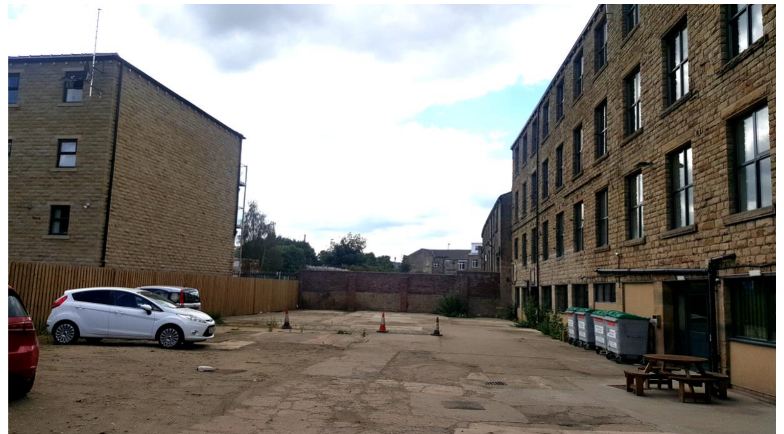
Fig 1: Existing site including rear elevation of Broomfield House
