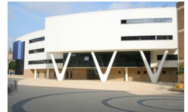
Fig 4: University of Huddersfield Creative Arts Building
